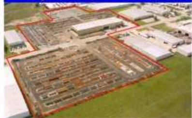
New Houston Warehouse
